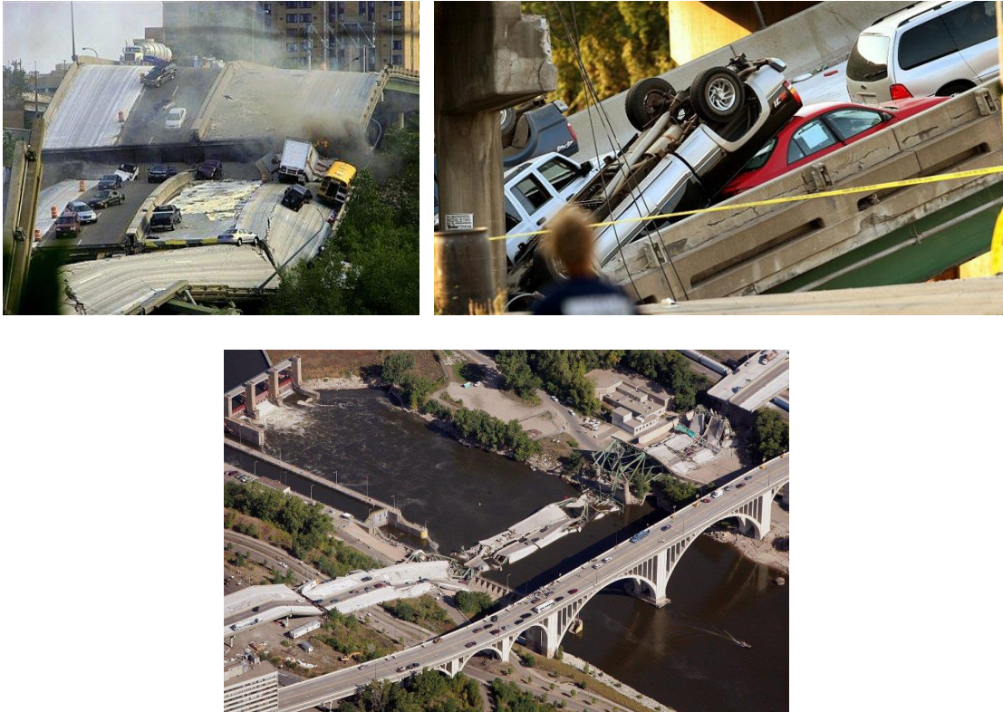
Figure 1. Collapsed 40 years old Minneapolis I-35W highway on the Mississippi River Bridge, August 1 st , 2007, killed 13 commuters and injured 145 motorists. A new bridge was built on the same spot at a cost of $250 million and reopened on September 18, 2008. The Federal Highway Administration (FHA) suggests that one in four of the more than 600,000 bridges in the USA are either "inadequate" or outdated.
