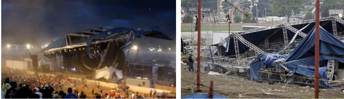
Figure 2. Collapse sequence of stand at the Indianapolis State Fair as a result of a storm wind gust, August 13, 2011 resulted in 5 casualties.
