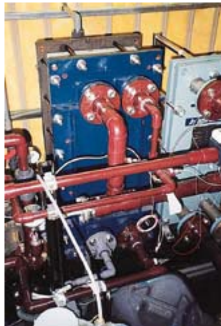
Figure 35. Hydrophobic Membrane Distillation operation and module developed by Takenaka, Japan.
