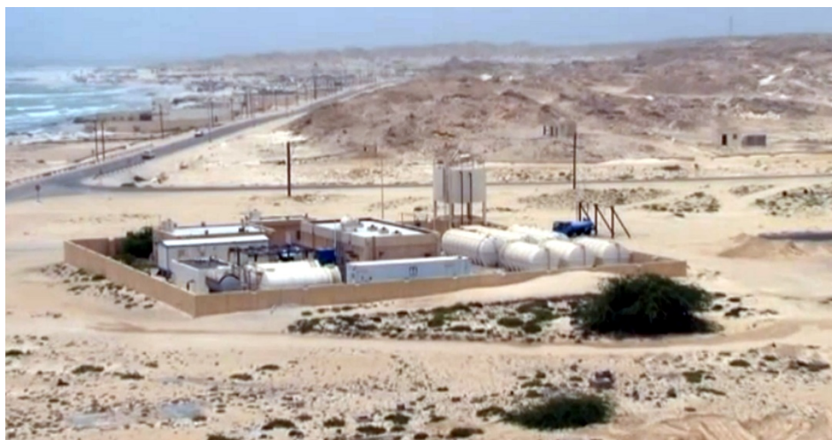
Figure 38. Al Khaluf Reverse Osmosis desalination plant, Gulf Coast. Source: Video clip, BBC.
