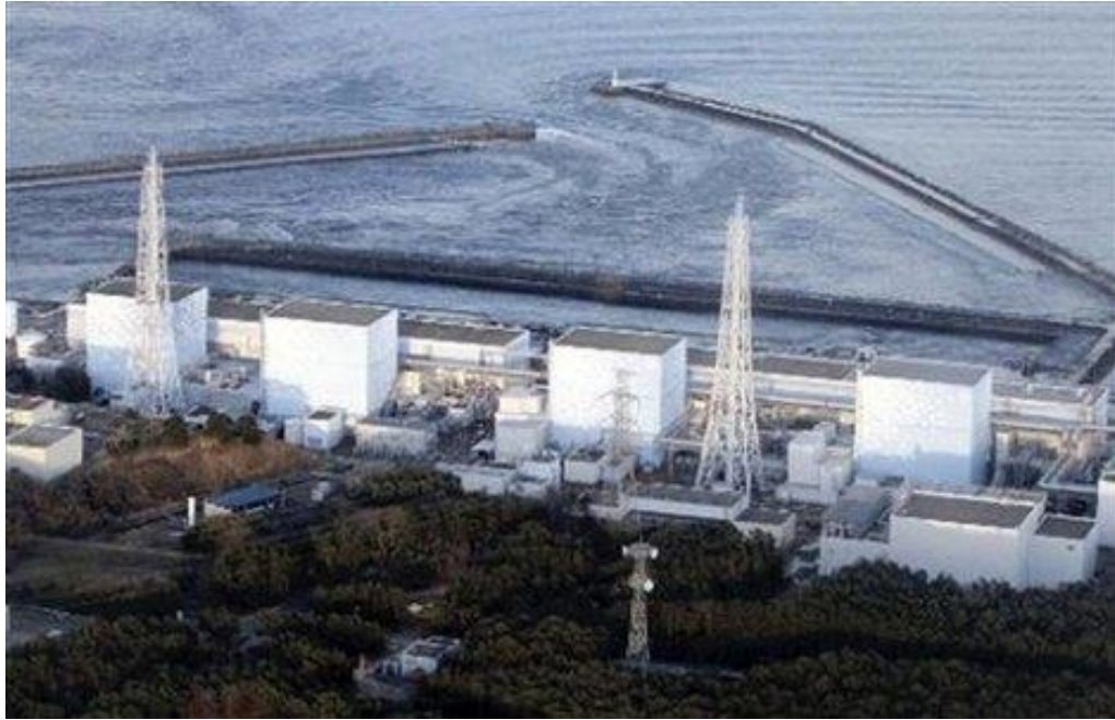
Figure 5. Siting of Fukushima plant down a hill sloping towards the sea. Source: Tepco.
