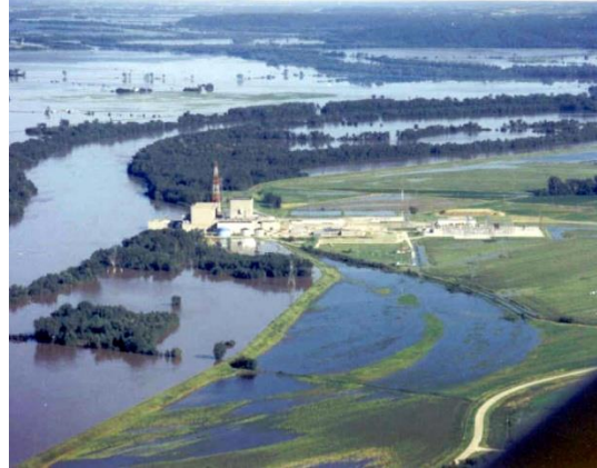
Figure 86. Cooper Station, Brownsville, Nebraska on the Missouri River flooding event, 1993.
