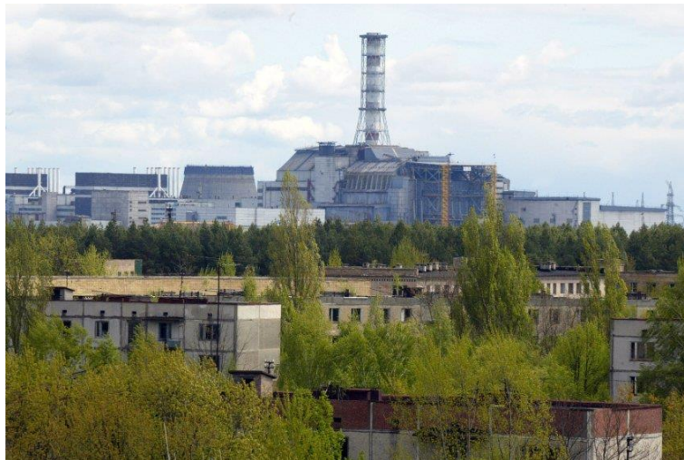
Figure 80. Encased damaged reactor at the Chernobyl site.
