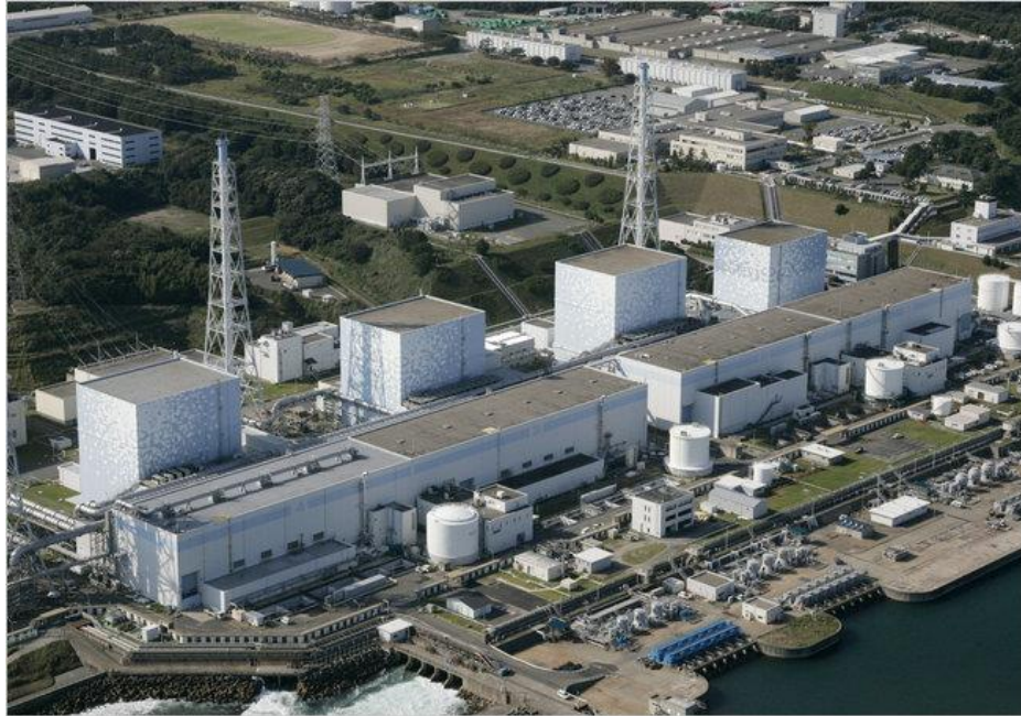
Figure 35. Fukushima Daiichi Boiling Water Reactors, BWRs nuclear Power plant, at Okumamachi, Fukushima Prefecture, Japan. The reactors are cooled with ocean water and are situated 148 miles or 238 km northeast of Tokyo. Connection to the grid shows up at the upper left side. Source: AP.
