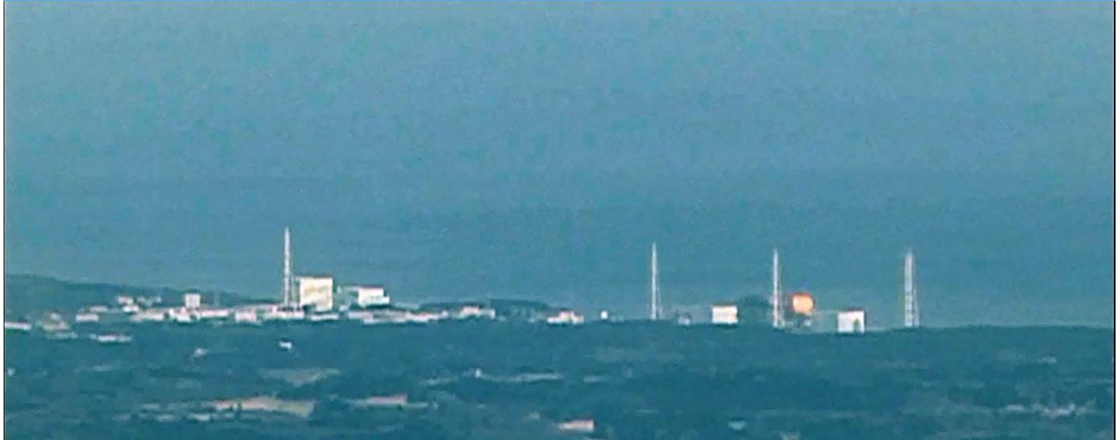
Figure 57. Lateral horizontally propagating hydrogen explosion at second chimney from the right preceded the vertical suspected steam explosion at unit 3.
