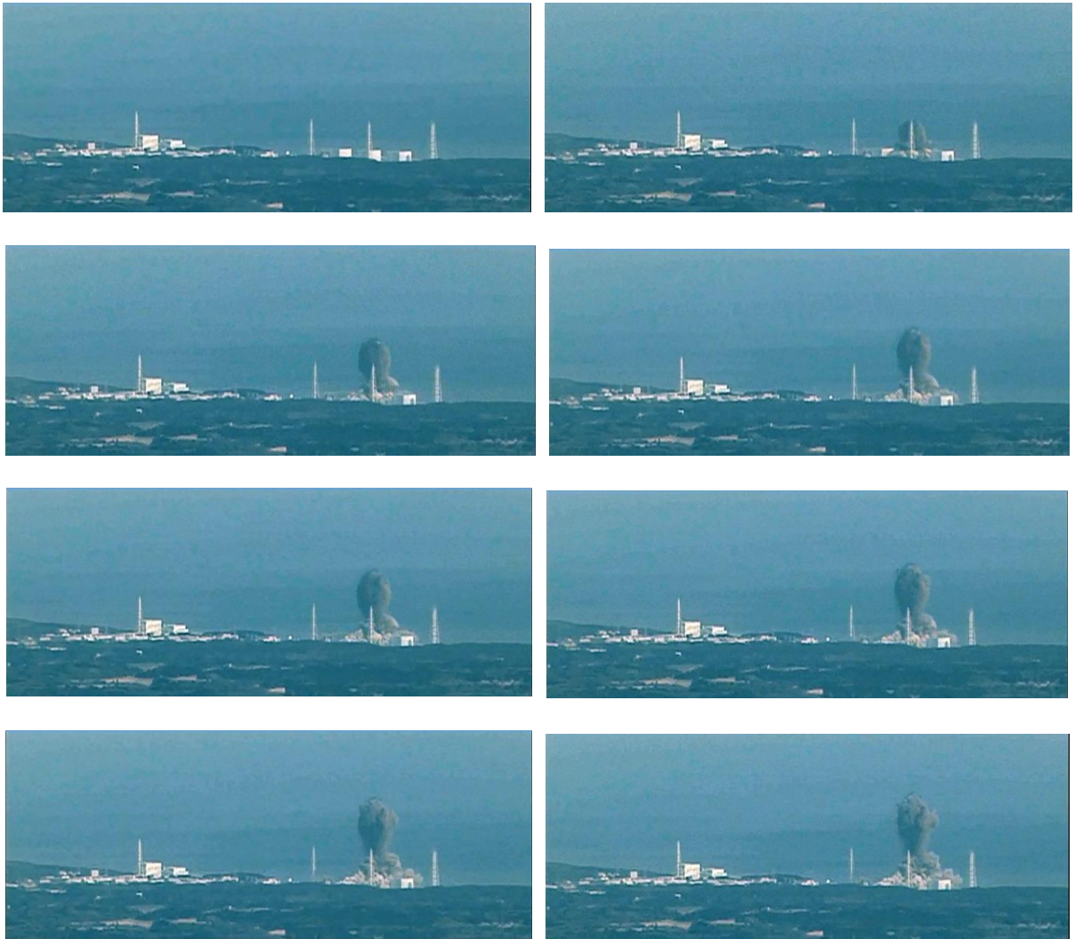
Figure 57. Lateral horizontally propagating hydrogen explosion at second chimney from the right preceded the vertical suspected steam explosion at unit 3.
