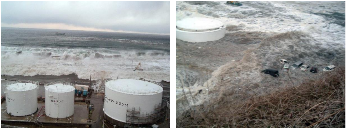
Figure 7 The tsunami wave more than 14 m (46 ft) high that originated 125 miles (200 kms) to the East, impinging on the 6 m protective wall and drowning the Fukushima Daiichi nuclear power plant site, March 11, 2011, Japan. According to the plant design, the maximum probable height of a tsunami at Fukushima was at just 5.7 meters compared with the actual 14 m. The breakwater wall offered protection against typhoons, but was breached by the tsunami. Source: Tepco.
