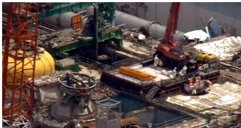
Figure 97. Extraction of fuel elements from fuel pool of unit 4.
