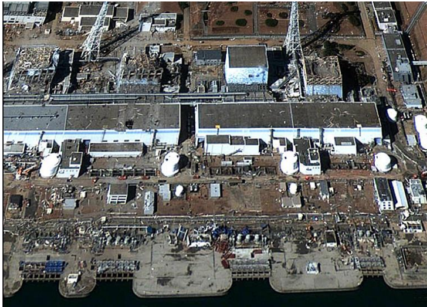
Figure 78. Aftermath of Fukushima Daiichi accident on March 11, 2011, one week after the accident. Rubble from hydrogen explosions in units 1, 3 and 4 and fire in unit 3 is spread over the site. Damage from earthquake and tsunami to the electrical systems apparent along the water front. Steam still emanating from unit 2. Source: Digital Globe.
