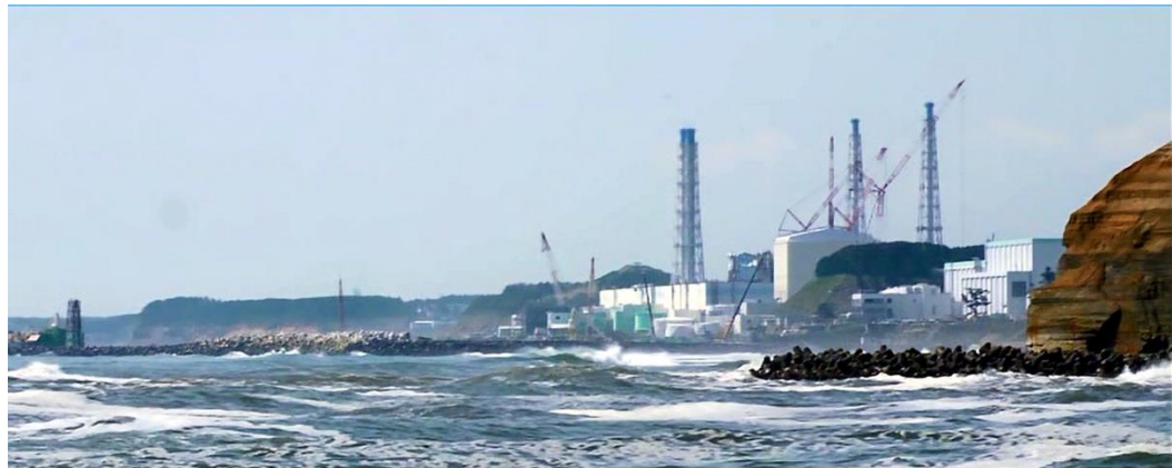
Figure 6. Siting of Fukushima plant on an artificially flattened area close to sea level. Source: Tepco.
