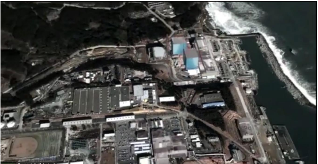
Figure 8. Units 5 and 6 were constructed on high ground by the General Electric and Ebasco Companies and were not affected by flooding and remained intact.
