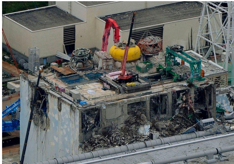
Figure 96. Debris and fuel elements removal from fuel storage pools at Fukushima.
