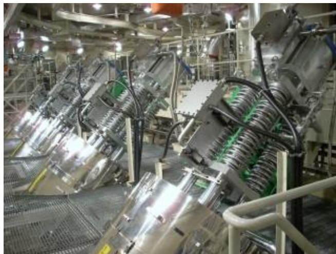
Figure 15. BWR Main Steam Isolation Valves, MSIVs. Source: Tepco.
