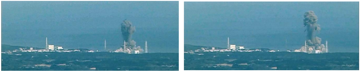
Figure 58. Sequence of vertical steam explosion following the horizontal hydrogen explosion at unit 3.
