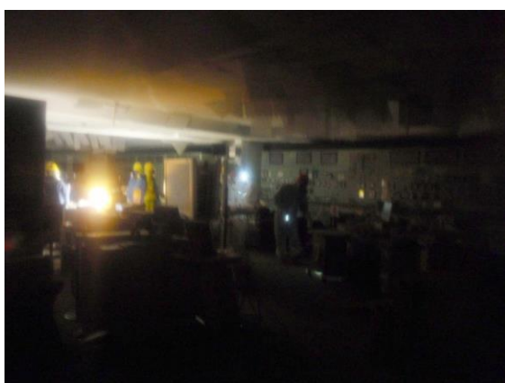
Figure 32. Station Blackout loss of power to the control room of the Fukushima Daiichi unit 1 reactor on March 24, 2011. Restoring offsite power to units 1 and 2 and power to the control room of unit 2 on March 26, 2011. The hanging ceiling tiles resulted from the earthquake. Source: Tepco.
