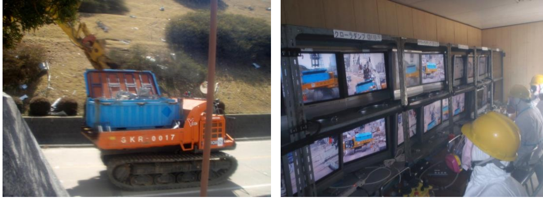
Figure 82. Removal of debris using remote control equipment and autonomous transporters. A useful design feature at the Fukushima site is an emergency command control center in an earthquake proof bunker with power supplies, radiation shielding thick walls, communication gear, food and water supplies and two air filtration systems. Source: Tepco.
