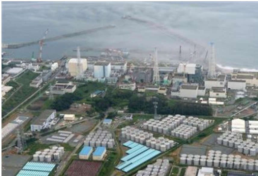
Figure 91. Liquid storage tanks at Fukushima.
