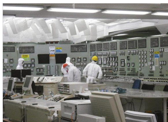
Figure 32. Station Blackout loss of power to the control room of the Fukushima Daiichi unit 1 reactor on March 24, 2011. Restoring offsite power to units 1 and 2 and power to the control room of unit 2 on March 26, 2011. The hanging ceiling tiles resulted from the earthquake. Source: Tepco.
