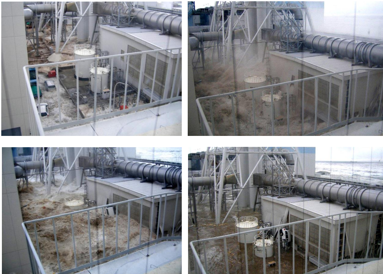
Figure 12. Fukushima Daiichi Tsunami water ingress and egress, drowning plant components at the base of the ventilation stack system, March 11, 2011. Source: Tepco.
