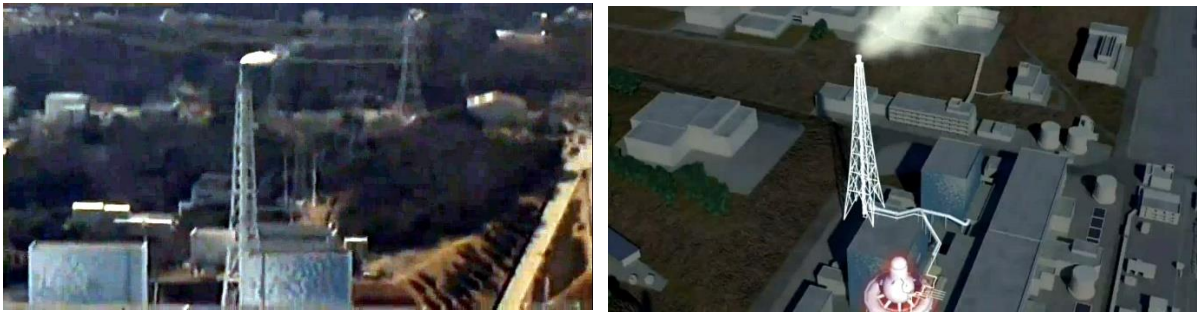
Figure 17. Venting primary containment of unit 2.
