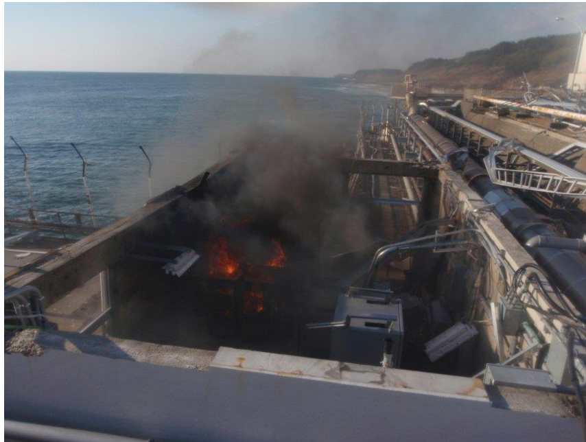
Figure 70. Fire in a battery bank initiated by a 6.3 scale aftershock on April 12, 2011. Source: Reuters.
