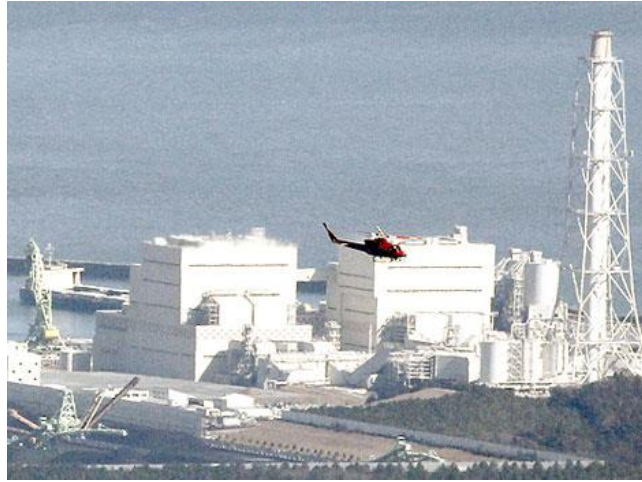
Figure 16. Steam appears to be leaking from top of left containment structure prior to hydrogen explosion. Source: Reuters.
