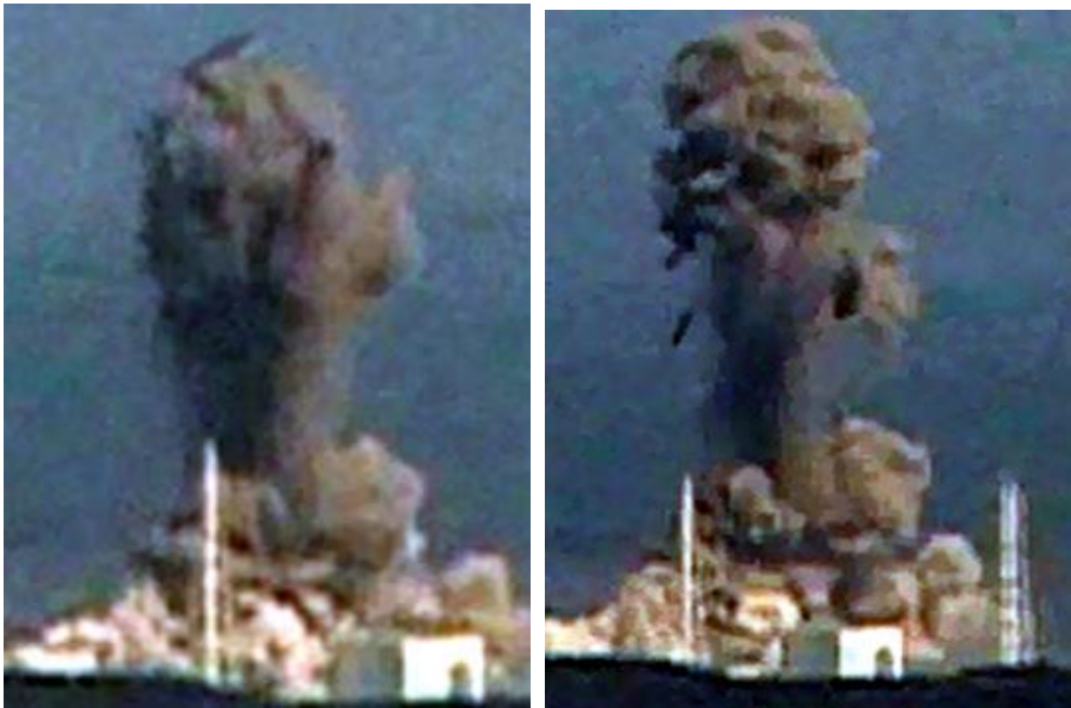
Figure 59. Highly energetic vertically propagating hydrogen or possibly steam explosion at the Fukushima Daichi unit 3 BWR on March 14, 2011 was followed by a fire and reactor fuel damage. Heavy debris possibly composed of the concrete shield plug or crane components was vertically ejected and is seen falling back down in the photograph. No damage to the reactor vessel can be inferred from the absence of the reactor's top plug in the ejecta. It bears some analogy to the complex aerodynamics of an "exploding vortex ring." Sources: NTV / NNN, Japan.
