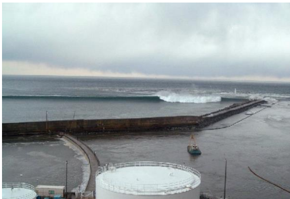
Figure 6. Siting of Fukushima plant on an artificially flattened area close to sea level. Source: Tepco.
