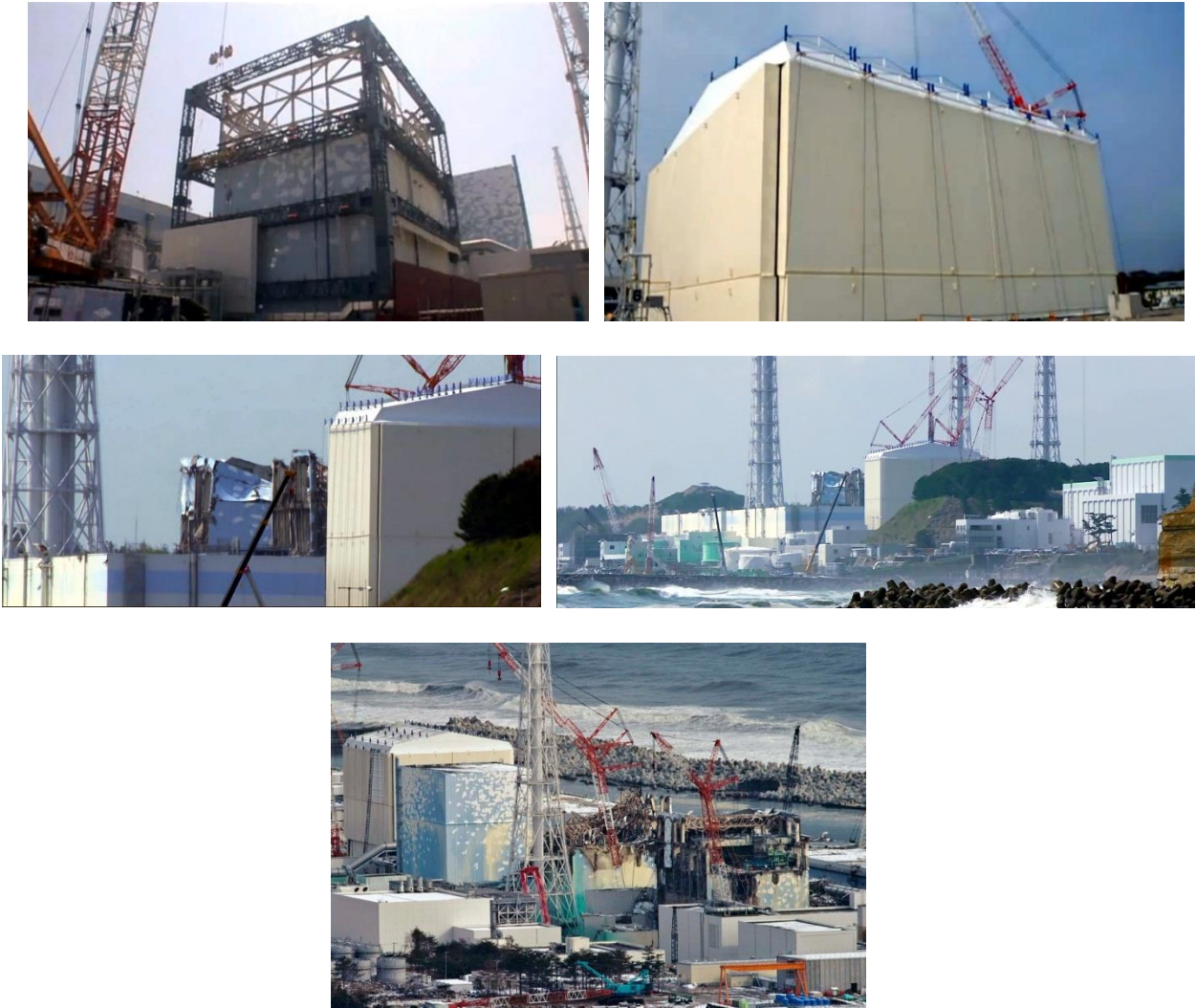
Figure 81. Cocoons encasing the damaged Fukushima reactors.
