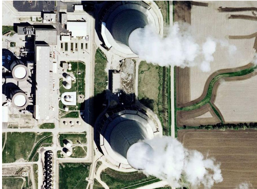
Figure 68. Steam generation from the twin cooling towers of the Byron nuclear power plant, Illinois, USA. The two reactor units are the smaller circular structures at the far left. Photo: Microsoft Bing.
