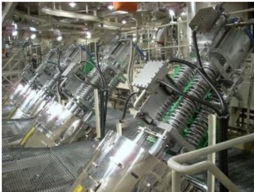
Figure 30. BWR main steam isolation valves.
