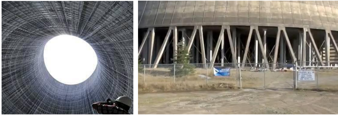
Figure 3. Interior and base view of cooling tower shell.
