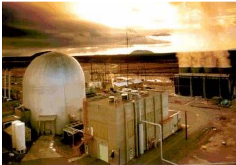
Figure 3. The Experimental Breeder Reactor II, EBR-II, at Idaho used a sodium coolant and operated for 25 years.
