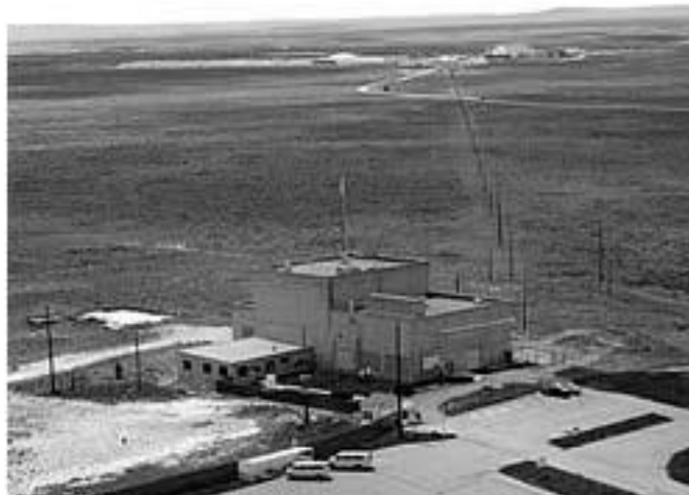
Figure 1. The Experimental Breeder Reactor I, EBR-I, in the Idaho desert turned into a museum. It used a Na-K eutectic alloy that was liquid at room temperature as a coolant.
