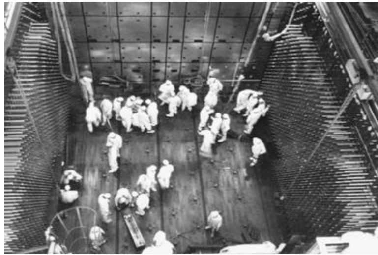
Figure 12. Assembly of the core of the C reactor at Hanford, state of Washington.
