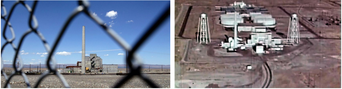
Figure 11. Views of the Hanford piles rising 120 feet above the desert floor with the water cooling treatment facilities, and the Columbia River in the background.
