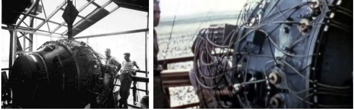
Figure 34. Photographs of the Trinity device on top and at bottom of its test tower showing the 32 initiators wiring.
