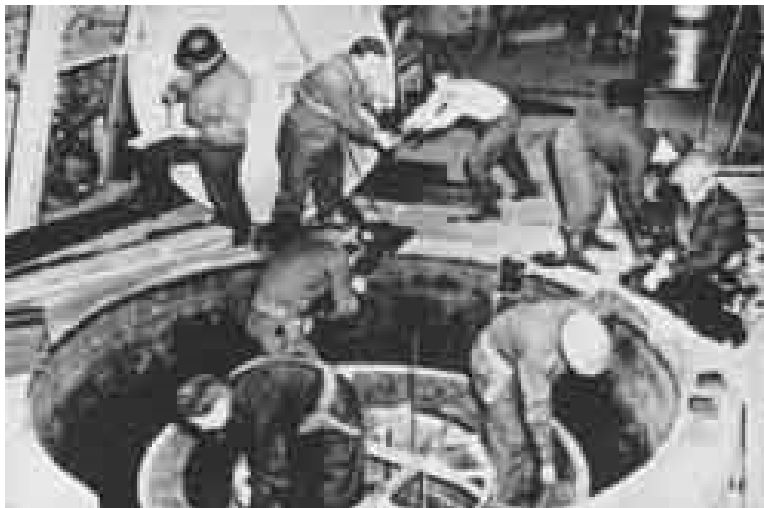
Figure 5. The Alsos team dismantling by hand the heavy water ( D_2O , HDO) subcritical assembly at the village of Haigerloch, Germany.
