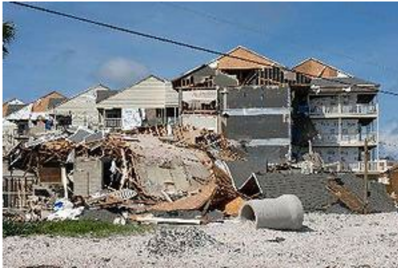
Figure 70. Damage to housing at Pensacola Beach, Florida from hurricane Dennis, July 16, 2005. FEMA photograph.
