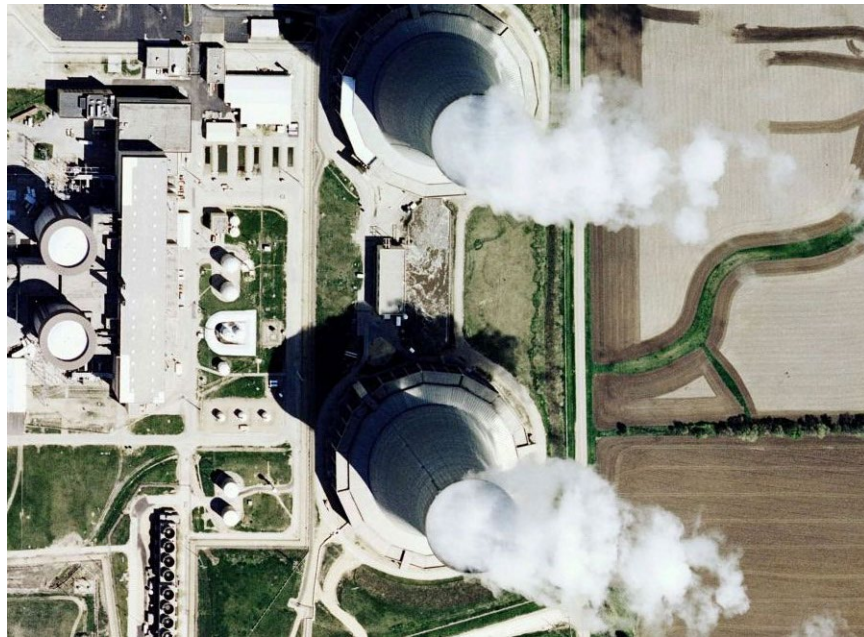
Figure 86. Steam generation from the twin cooling towers of the Byron nuclear power plant, Illinois, USA. The two reactor units are the smaller circular structures at the far left. Photo: Microsoft Bing.
