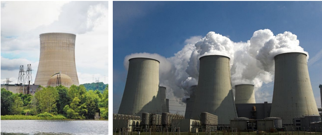
Figure 85. Cloud seeding from nuclear and fossil fuel power plants' cooling towers.
