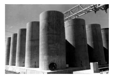
Figure 10. Concrete silos temporarily store the used fuel elements allowing cooling before final recycling or disposal.
