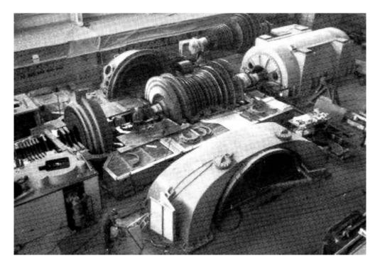
Figure 8. Electrical generator and disabled steam turbine in the Douglas Point plant.
