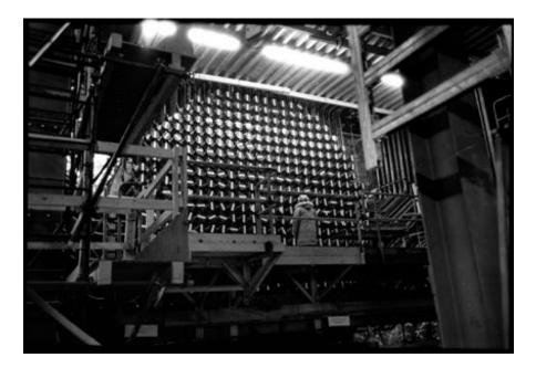
Figure 4. Darlington CANDU reactor face showing the horizontal pressure tubes.
