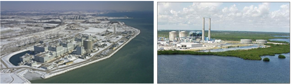
Figure 1. Darlington 935 MWe CANDU Heavy Water Reactor (top), and reactor complex at Ontario, Canada.
