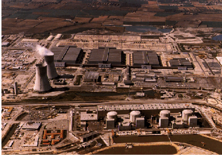
Figure 42. The Tricastin Gaseous Diffusion plant, France can provide enough enriched fuel for 90 power plants. Four nuclear reactors are used to supply it with its electrical needs.
