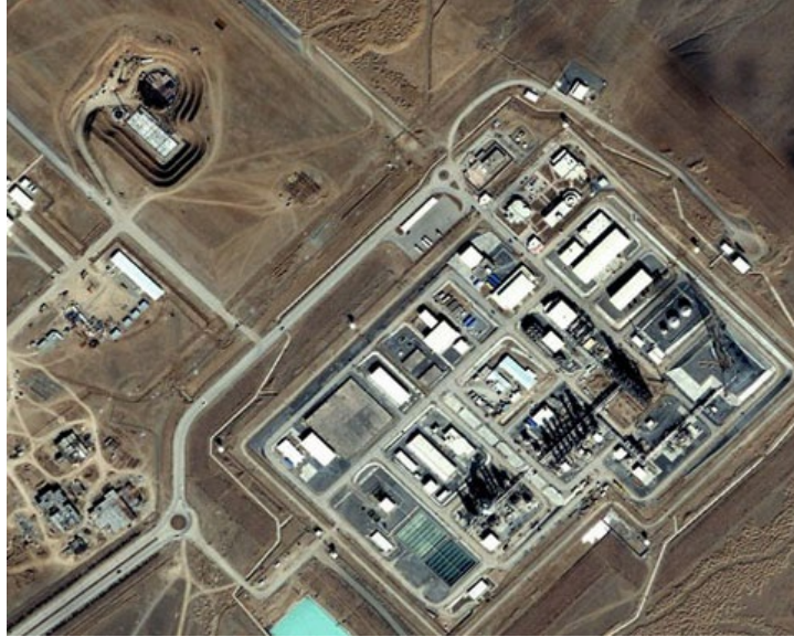
Figure 9. Arak, Iran heavy water production plant showing distillation towers, February 2005.
