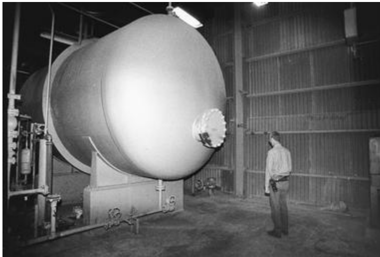
Figure 12. Lithium solution tank used in the COLEX process. The \text{Li}^6 can be separated from the amalgam and the tailings fraction of \text{Li}^7 is electrolyzed from the aqueous solution of lithium hydroxide for further use.
