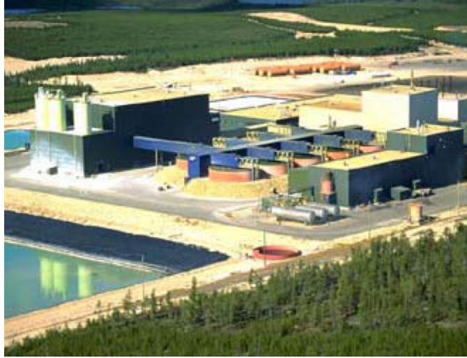
Figure 24. Uranium mill at Key Lake, Northern Saskatchewan, Canada. Source: Cameco.
