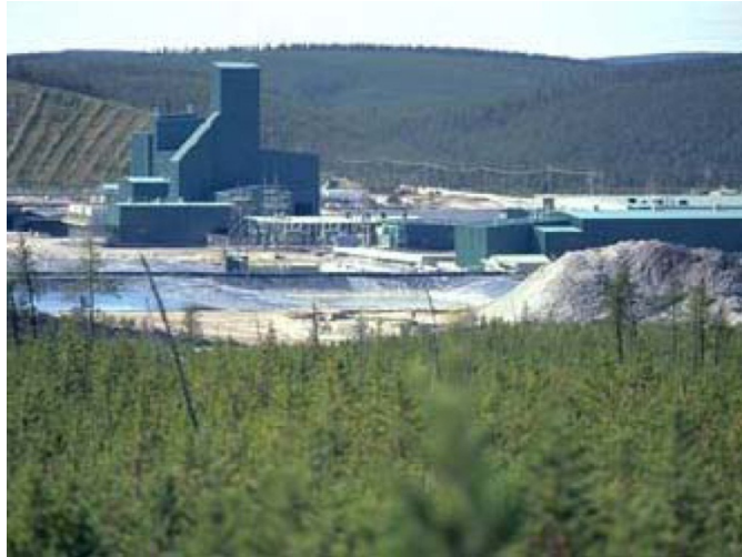
Figure 15. McArthur River Cameco underground uranium mine in Northern Saskatchewan, Canada.
