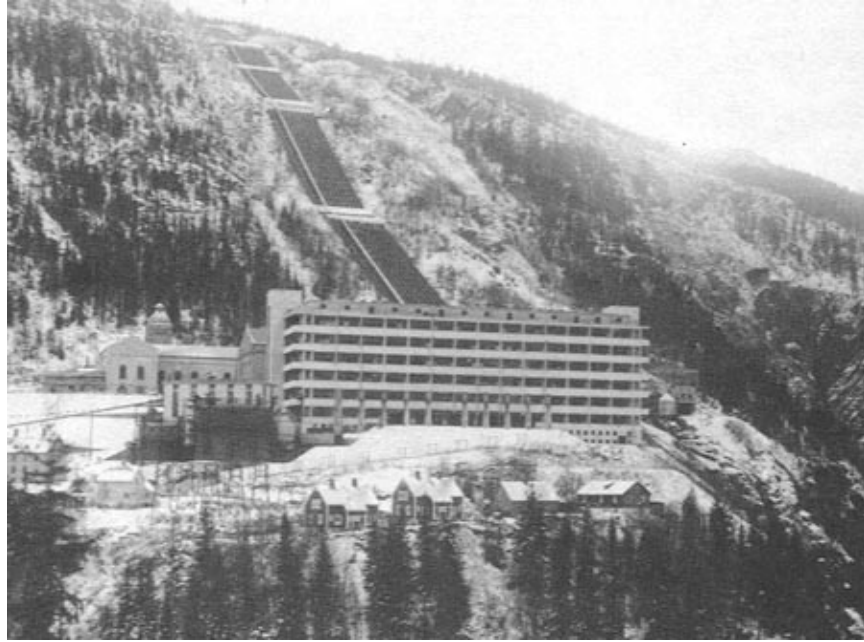
Figure 3. Norsk Hydro heavy water electrolysis production plant at Vemork, Norway.
