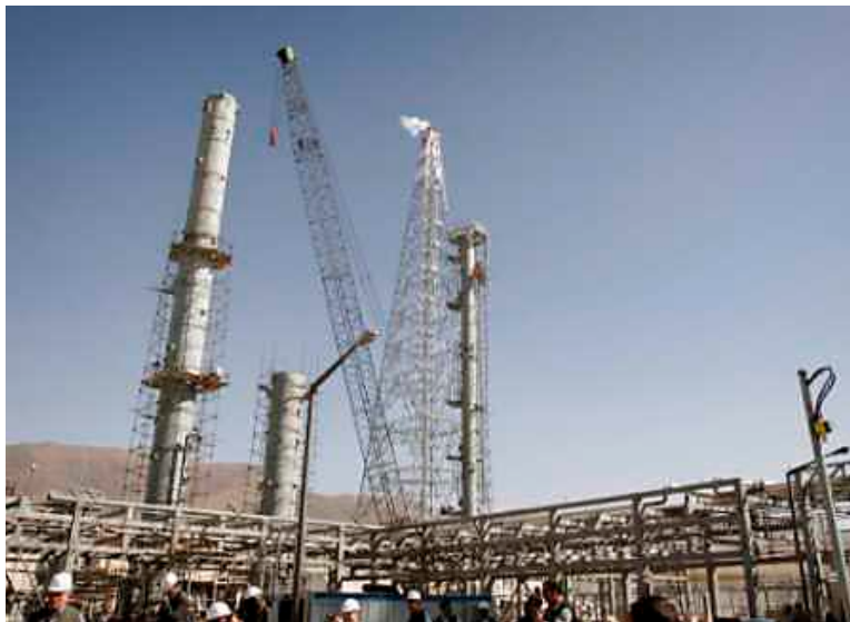
Figure 8. Arak, Iran heavy water plant under construction.
