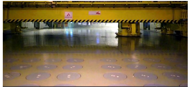
Figure 30. Storage wells for vitrified waste containers at the Marcoule plant in France.
