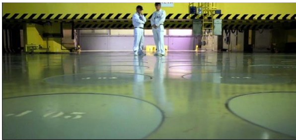
Figure 30. Storage wells for vitrified waste containers at the Marcoule plant in France.
