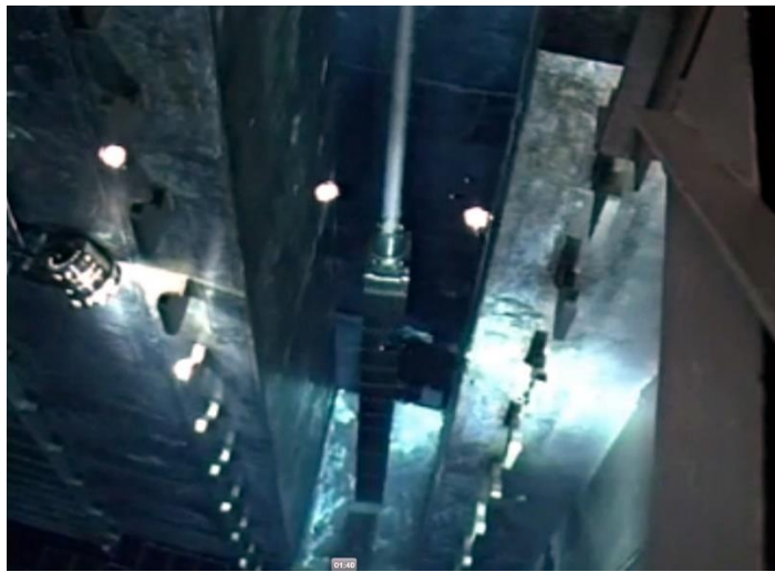
Figure 9. Fuel element storage in fuel storage pool.
