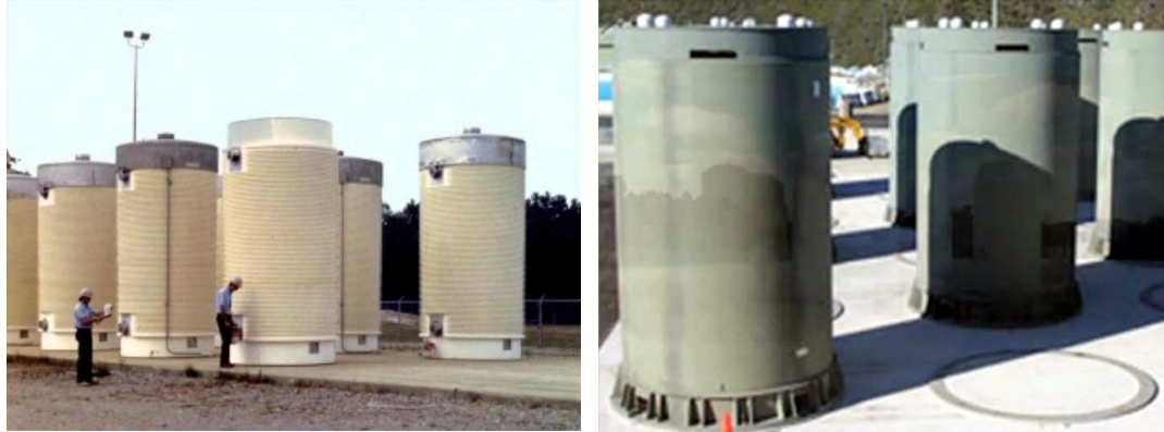
Figure 38. Outdoor dry storage silos at nuclear power plants sites. Source: Ameren.
