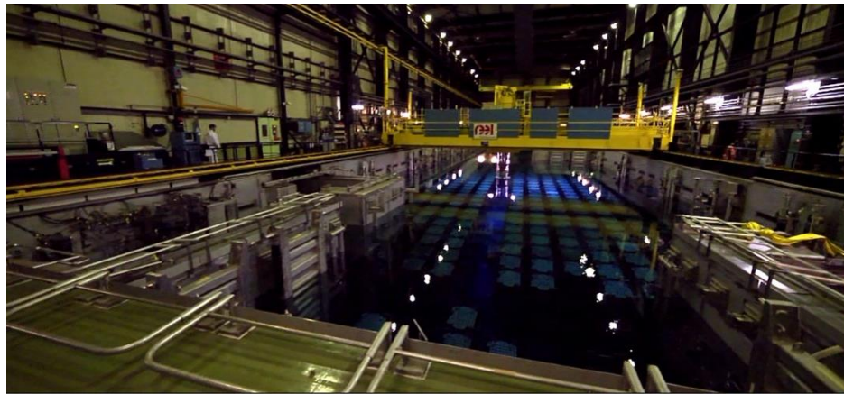
Figure 14. Fuel storage pool at reactor compound, France.
