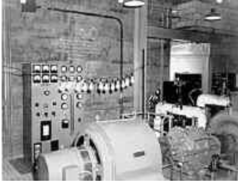
Figure 33. The Experimental Breeder Reactor I, EBR-I, lighted up a string of light bulbs with the first produced nuclear electricity on December 20, 1951.
