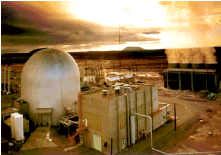
Figure 34. The Experimental Breeder Reactor II, EBR-II, at Idaho used a sodium coolant.
