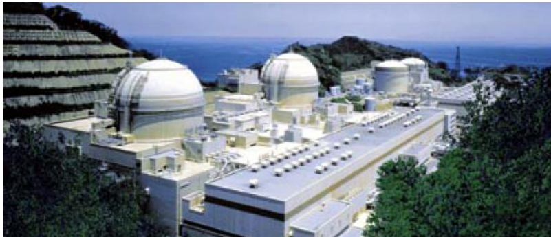
Figure1. Ohi power station complex, operated by Kansai Electric Power Inc., Japan.
