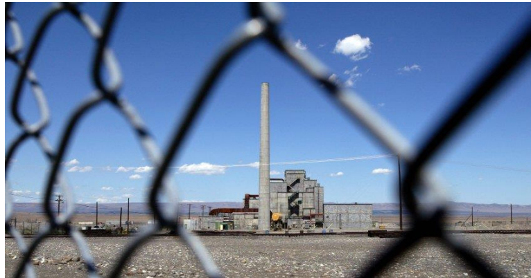
Figure 34. Decommissioned B Reactor at the Hanford reservation site is open for visitors as a historic national landmark, Washington, USA.
