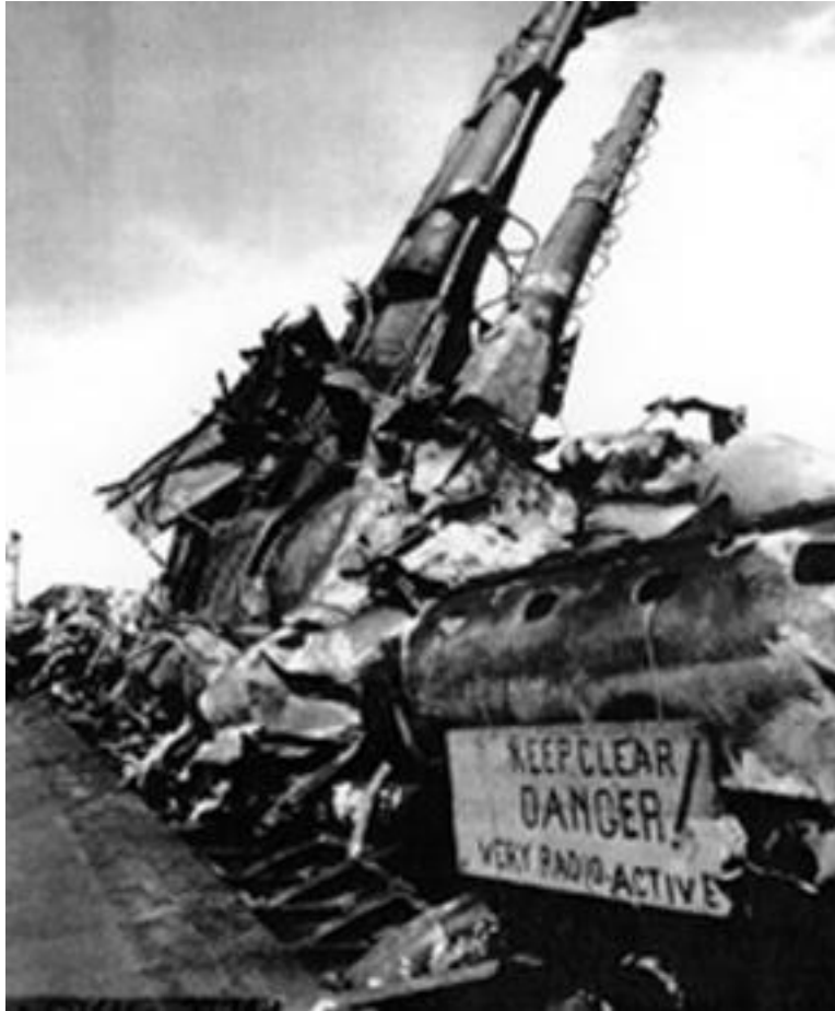
Figure 8. Severe damage to the USS Skate, Able test, operation Crossroads, July 1 st , 1946.
