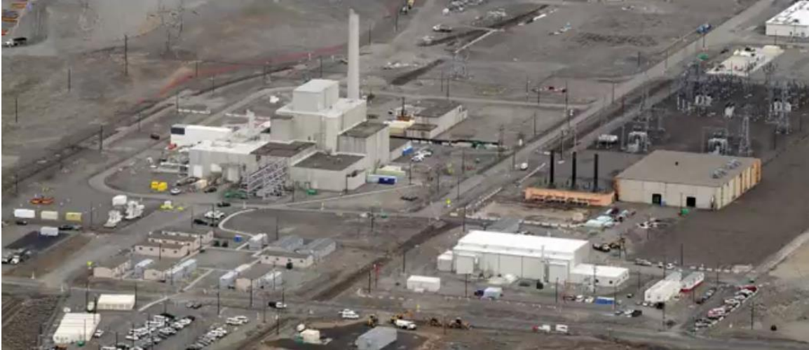
Figure 35. Reactor site with associated auxiliary buildings and electrical switchyard.
