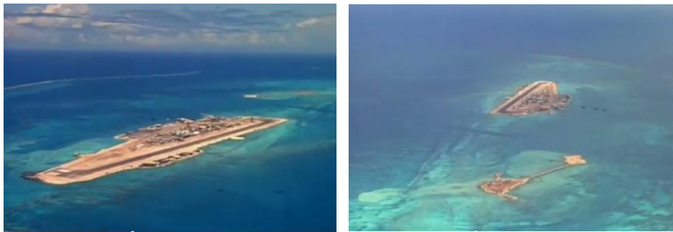
Figure 30. Johnston Island proving grounds facilities.
