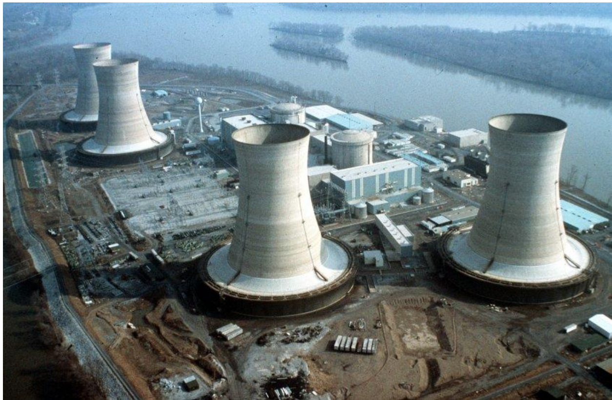
Figure 1. Metropolitan Edison's unit 2 Pressurized Water Reactor (PWR) of 961 MWe of electrical capacity is the capped cylindrical building between its two cooling towers in the foreground. Unit 1 in the back was unaffected by the accident and continued operation.
