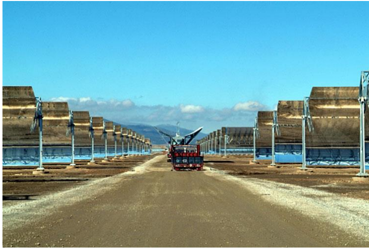
Figure 36. Andasol 1 plant, Solar Millenium, Spain.
