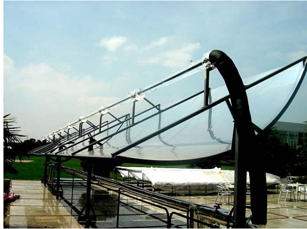
Figure 5. Captain John Ericsson longitudinal trough parabolic concentrator with a steam engine using a flywheel for energy storage, 1883 [15] (top), and its modern realization (bottom).
