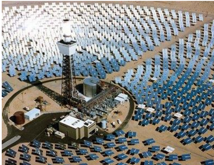
Figure 7. Central Receiver or Solar Tower plant.
