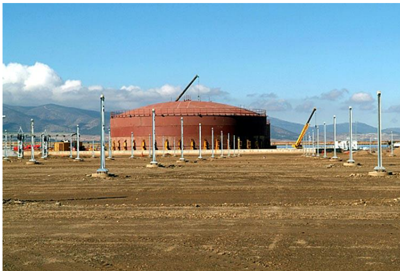
Figure 11. Molten Salt Thermal Energy Storage Tank for electrical power generation, Andasol 1 plant, Spain. Source: Solar Millenium.
