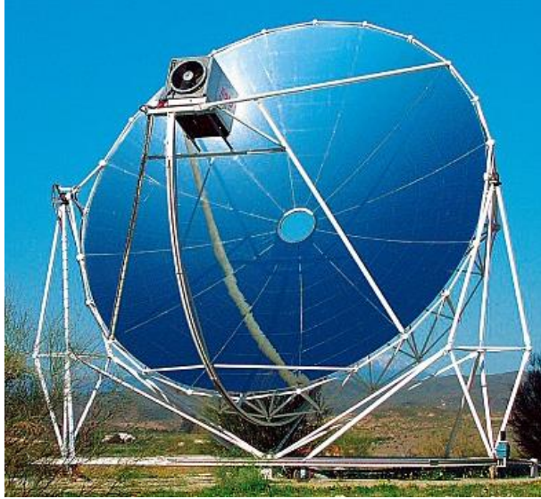
Figure 38. Plataforma Solar single dish associated with a Sterling engine system, Almeria, Spain.
