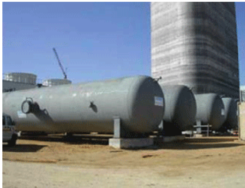
Figure 24. Evolution of experimental tanks to commercial storage tanks at the Andasol 1 and PS10 plants, Spain.
