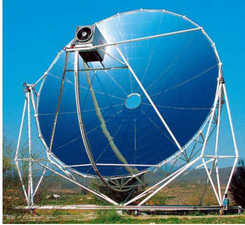
Figure 21. Solar dish concentrator, Plataforma Solar, Almeria, Spain. The concave mirror concentrator focuses solar radiation on a Stirling engine receiver using He as a working medium. Source: Der Spiegel.
