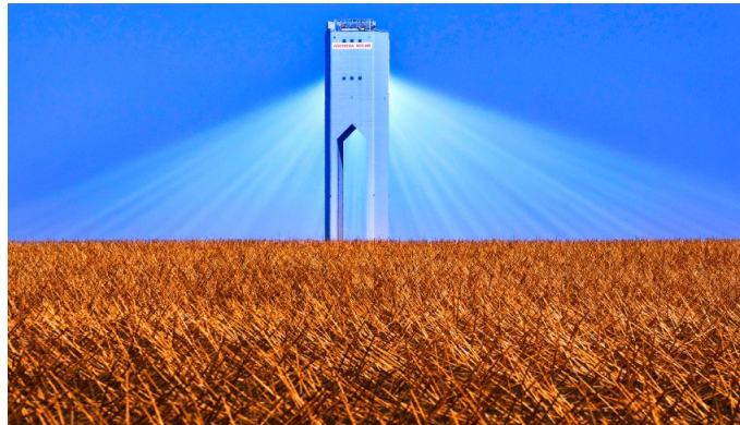
Figure 14. The PS20 Solar Power Tower is the world's largest, Andalusia, Spain. Mirror array concentrates solar radiation on an absorber at the top of the tower with water and steam as working media. The tower supplies the energy need of 10,000 homes. Source: Der Spiegel.
