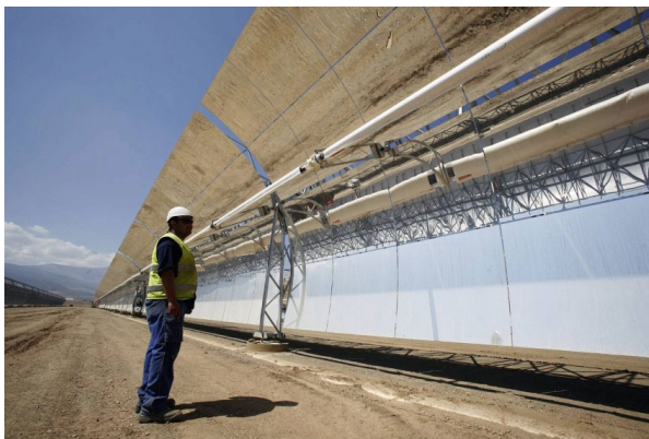
Figure 12. Andasol 1 solar plant in Grenada, Spain. The design follows the same principle of a solar plant built in Egypt 100 years ago; producing steam fed to a turbine running irrigation pumps for Nile River water. Source: DDP.
