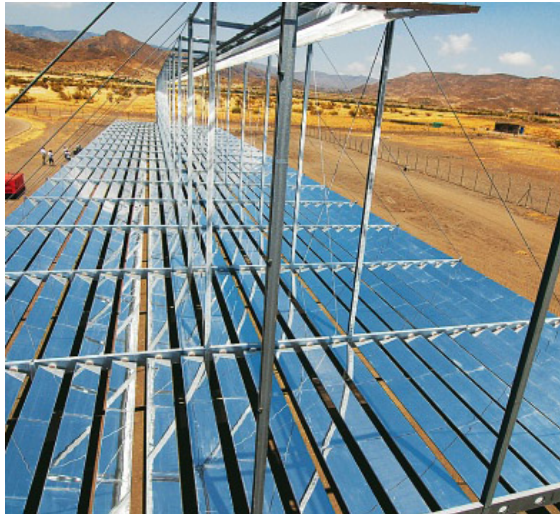
Figure 22. Fresnel lens mirror concentrator at Plataforma Solar, Almeria, Spain. Flat mirrors track solar radiation and focus it on a tube. The design is simpler and more economical than a trough concentrator but operates at a lower efficiency than a trough design. Source: Der Spiegel.
