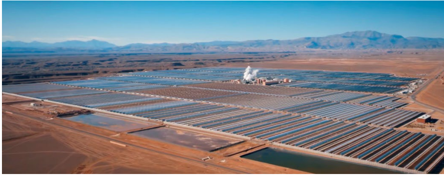
Figure 8. Nour (Al Nour: The Light, in Arabic) solar plant stores energy in Molten Salts at 400 degrees Celsius produces power for 3 hours after sunset from parabolic reflectors in the Sahara Desert at Morocco. Hydrogen as an energy carrier can be produced for export for fuel cell applications. Electricity can be produced for long distance high voltage DC (HVDC) power transmission.
