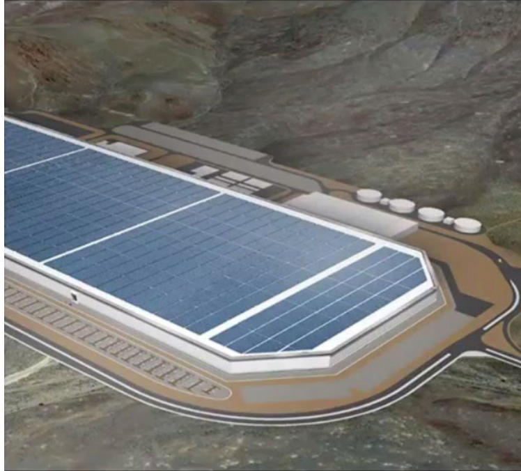
Figure 13. Gigafactory1 solar-powered battery manufacturing facility in Nevada, USA. Source: Tesla Power.
