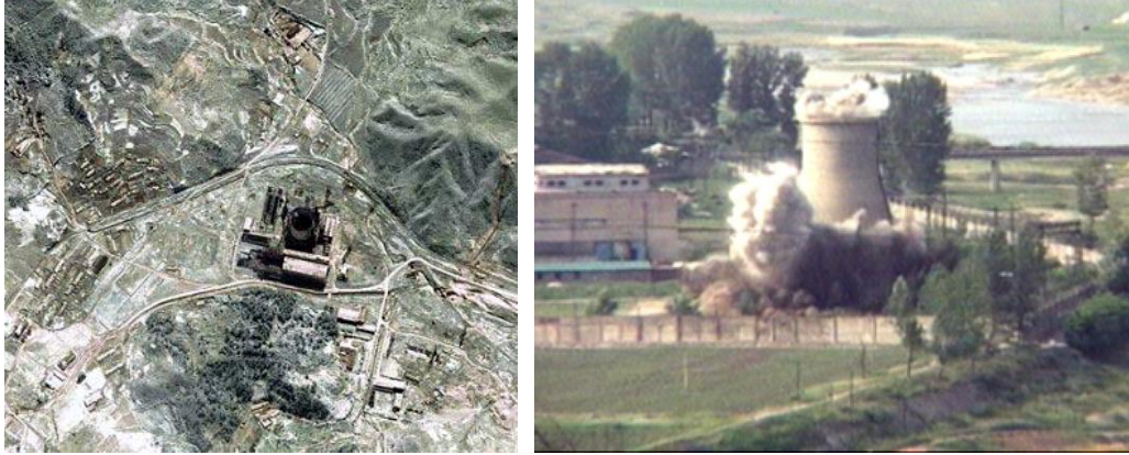
Figure 8. Aerial photograph of the Taechon 200 MWe power reactor under construction and the Yongbyon 1, 5 MWth research reactor in the DPRK. The cooling tower that appears to have been demolished in 2008 as a result of agreements was being reconstructed in 2013.
