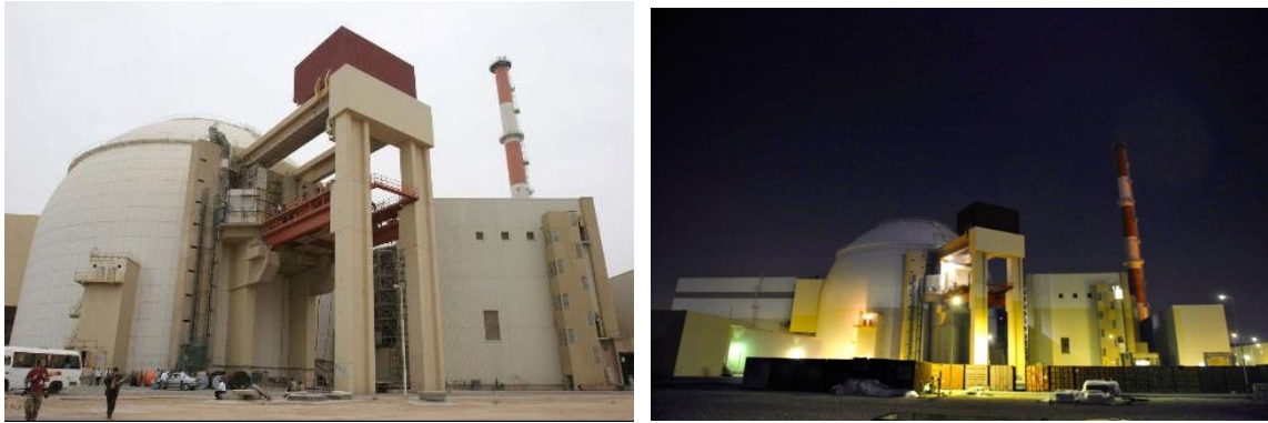
Figure 27. The Nuclear power plant at the port of Bushehr, Iran, under different stages of construction.
