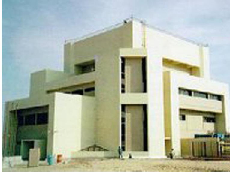
Figure 18. Exterior of the Egypt Research Reactor ETRR-2, 22 MWth research reactor at Inshass, Egypt.
