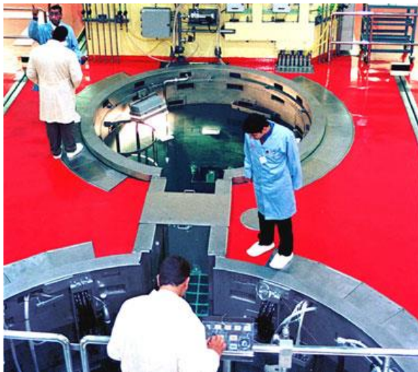
Figure 19. Interior views of the ETRR-2, open pool type 22 MWth research reactor at Inshass, Egypt.
