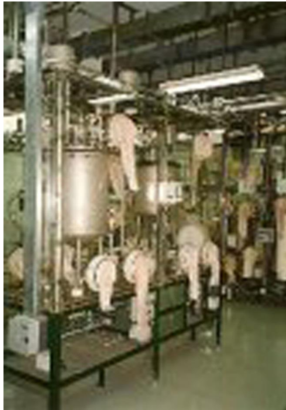
Figure 20. Fuel Manufacturing Pilot Plant (FMPP), Egypt.
