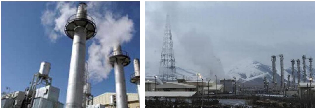
Figure 26. Heavy Water plant distillation towers at Arak, IRI.
