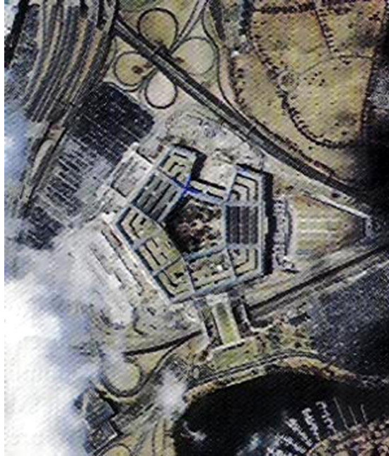
Figure 59. A one-meter resolution photograph taken by the Ikonos satellite showing a wing under reconstruction at the Pentagon building.
